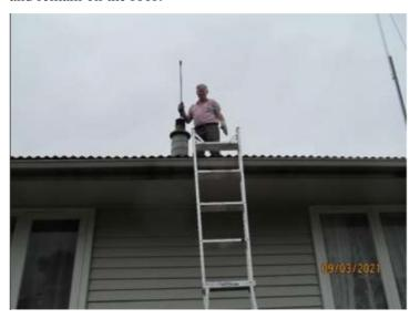
After two years use, the chimney flue had only a light powder that easily fell away as the brush dislodged it. I did not see any sap or resin adhered to the sides. The wood I get from Wecks in Patumahoe is obviously just the right sort of firewood for this chimney.
